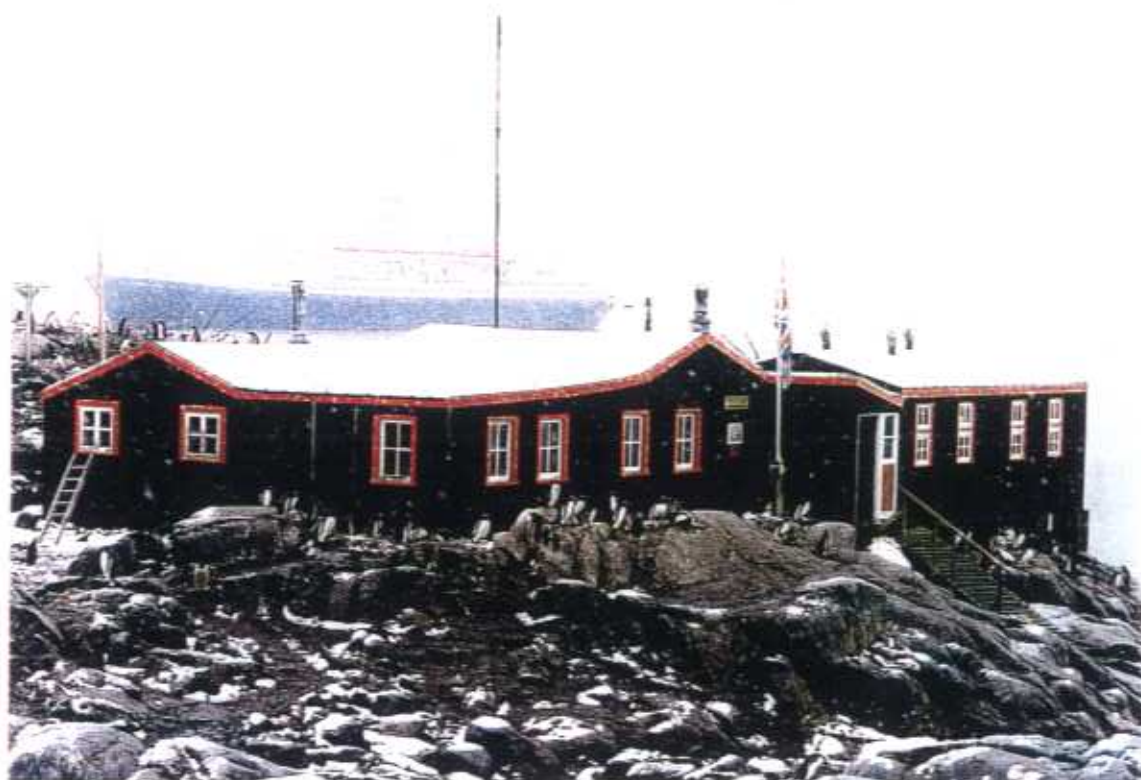
Bransfield House, Port Lockroy
