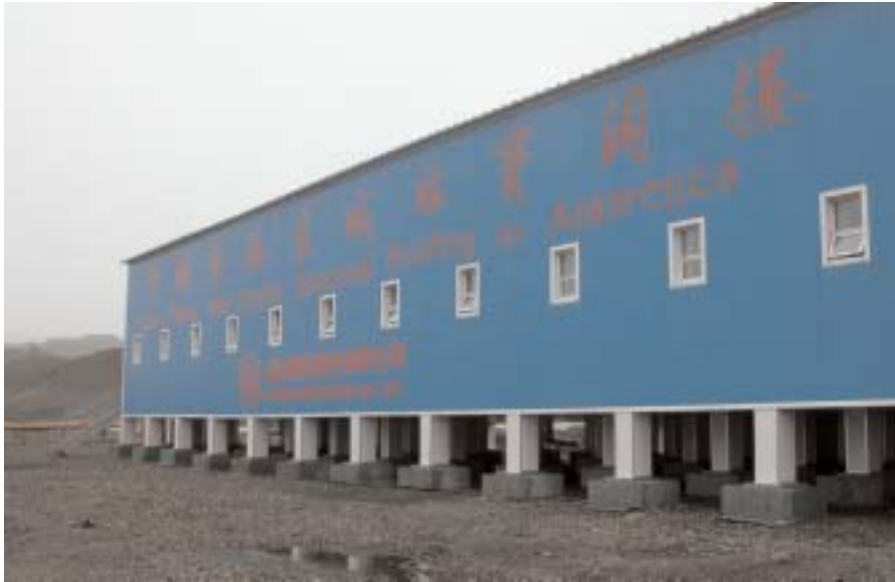
The recently constructed generator building.
