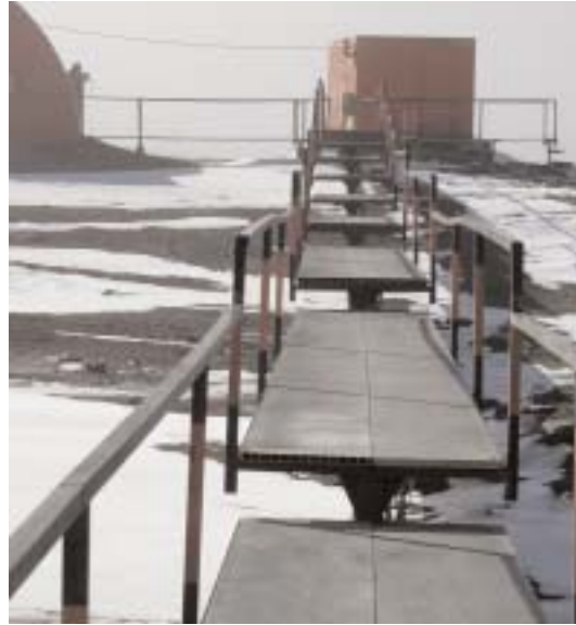
Elevated walkways which join all the station's buildings.
