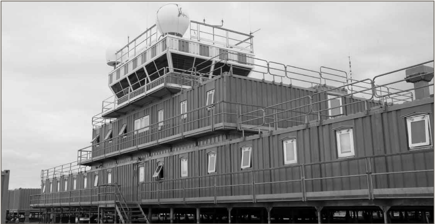
Mario Zucchelli Station Main Building
