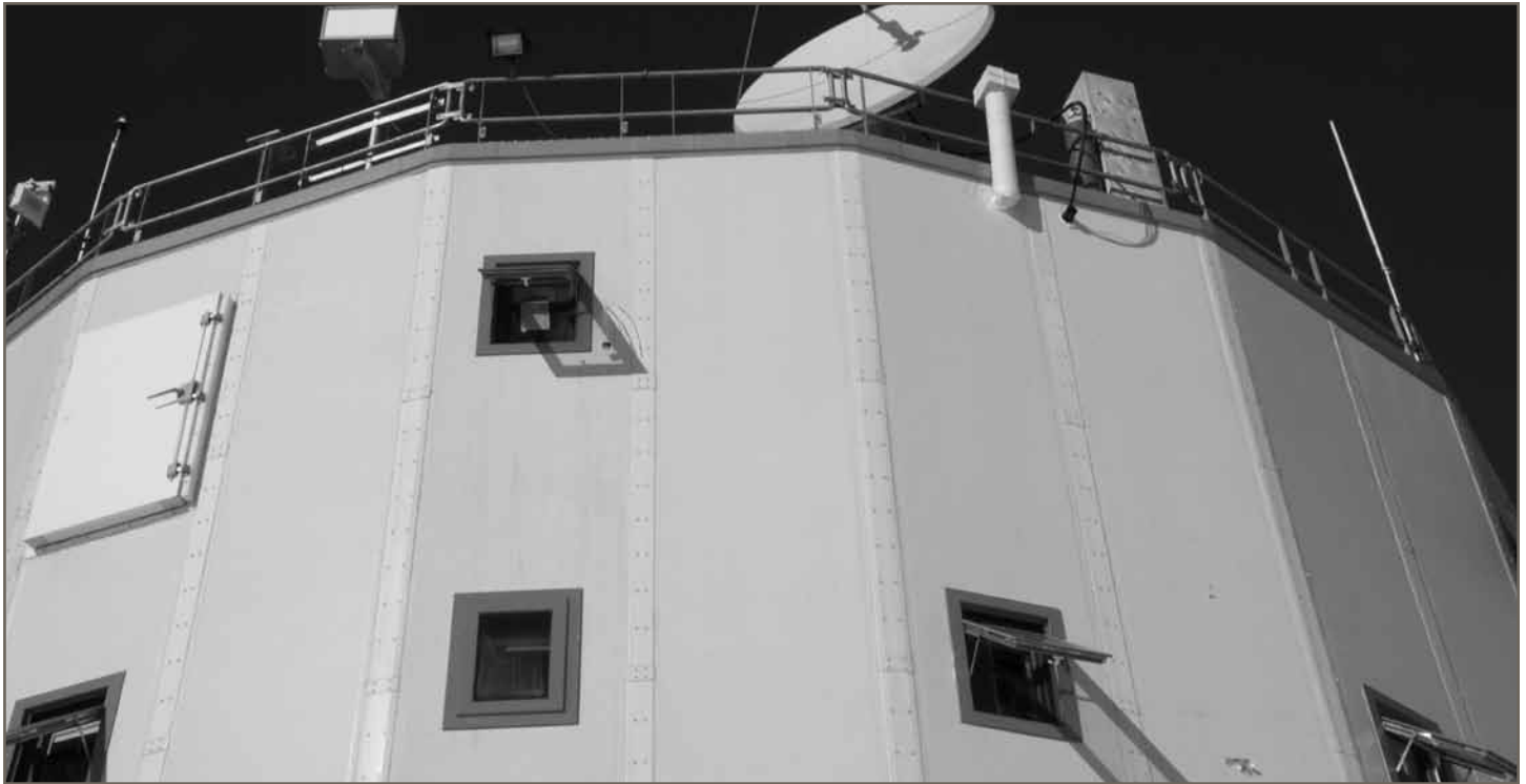
Open Exterior Windows at Concordia Station
