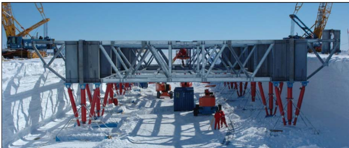
Garage structure with deck U1, bipod cylinders and foundation pads (Feb 2008)
